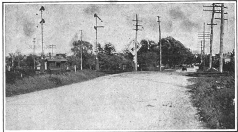
LOOKING TOWARD CROSSING IN DIRECTION AUTOMOBILE WAS TRAVELING.
